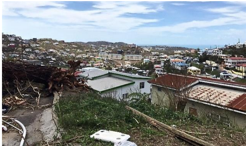
Figure 4.12: Annas Rest, with the damaged Tutu Hi-Rise apartments toward rear of the photo in St. Thomas. (James Gardner of the St. Croix Source, September 15, 2017)
