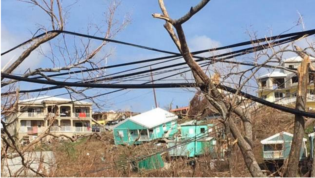
Figure 4.16: Hurricane Irma leaves debris and destruction in its wake on St. John, part of the U.S. Virgin Islands (Anthony Faiola / The Washington Post, 2017)
