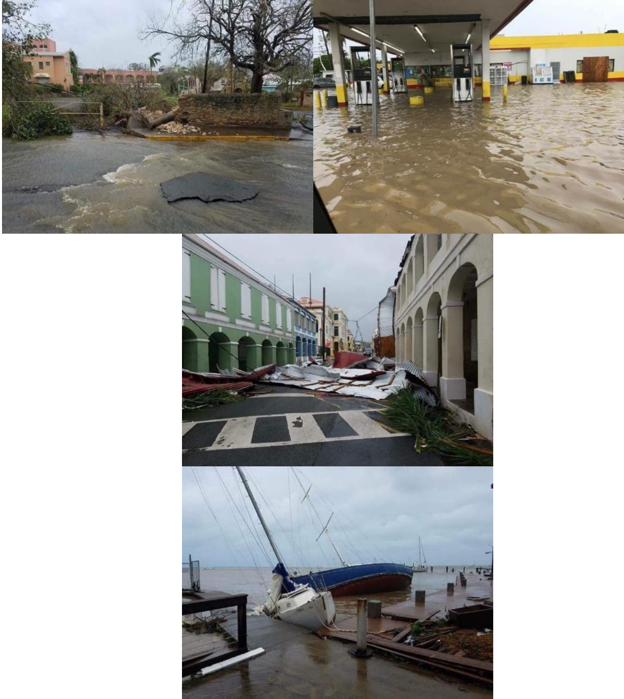
Figure 4.20: Damaged Infrastructure and Flooding in St. Croix Following Hurricane Maria
