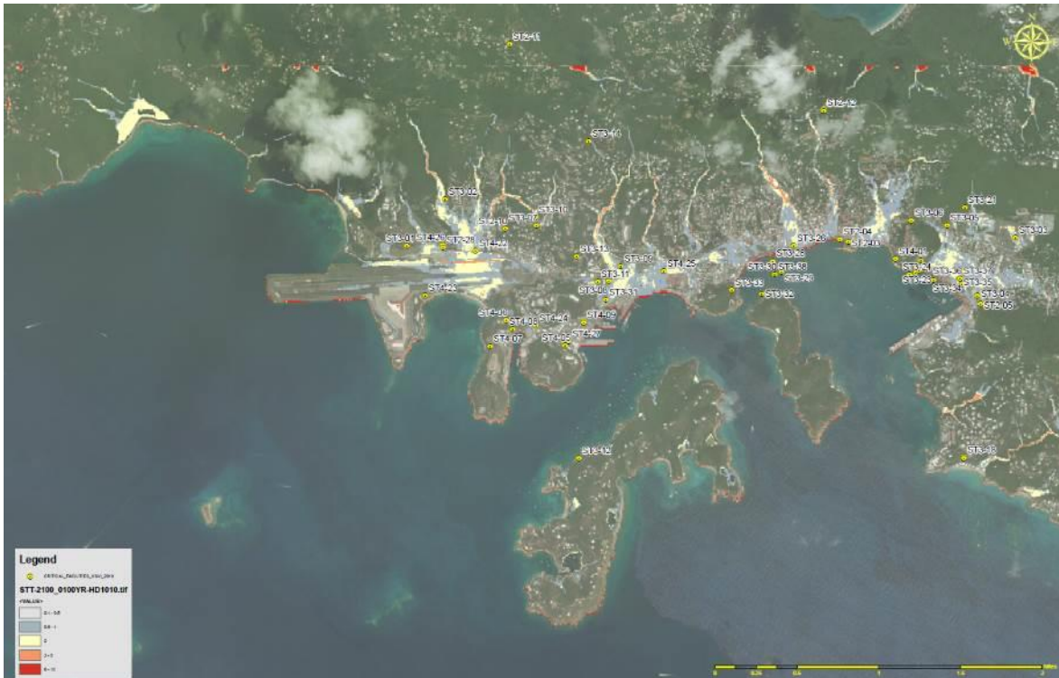
Figure 6.17: Flood Depth Analysis of 100-year 72-hour storm event for year 2100. The aerial shows the topography and computed depth of water (Appendix A13.MAP_STT_2100_0100_HD.pdf provides a higher resolution map)
