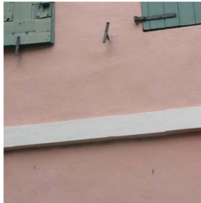
Fig. 10.706.40 – Masonry faced with Stucco
