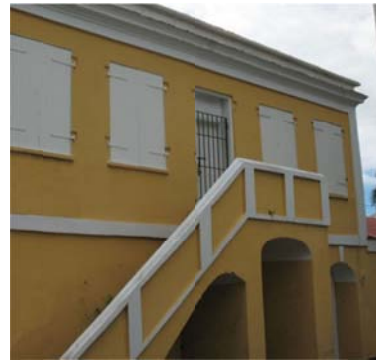
Fig. 10.706.27– Dog-leg with landing
