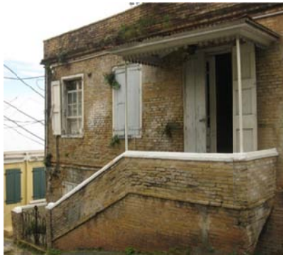
Fig. 10.706.26 – Dog-leg with landing
