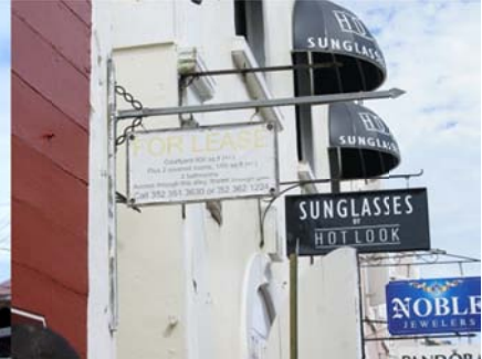
Fig. 10.705.33 – Sign mounted perpendicular to building façade.
