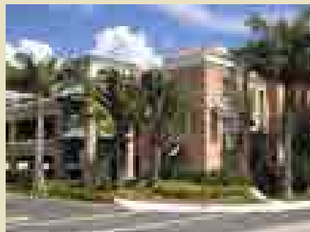
A liner building separates the garage from the street. (Mizner Park, West Palm Beach, FL)
