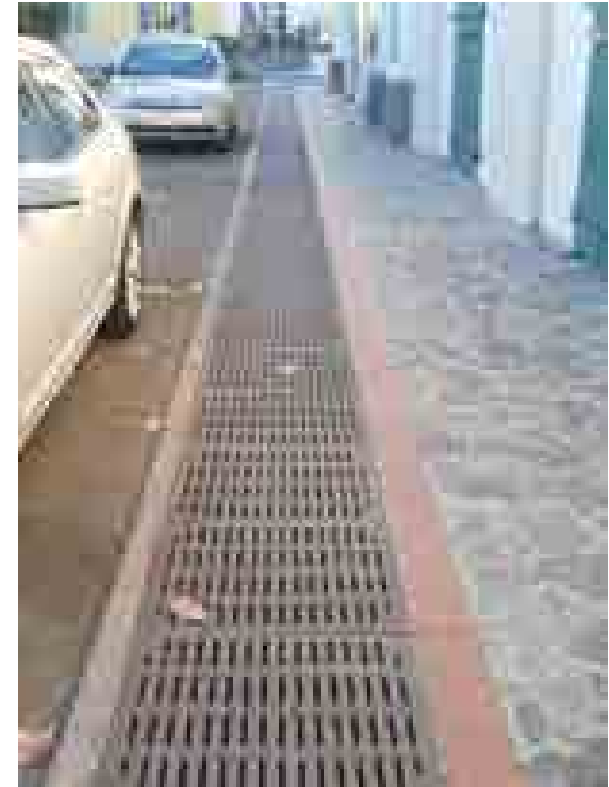
Drainage grates can be used to provide refuge area for pedestrians to step out of travel lanes.
