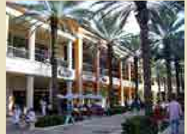
Street-oriented buildings coupled with new pedestrian amenities such as a wide sidewalks, street trees, and on-street parking create a walkable neighborhood center.
