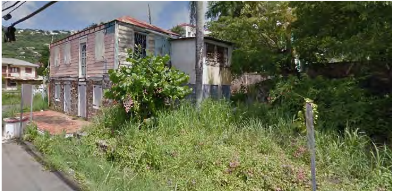
An overgrown lot adjacent to a building in need of rehabilitation. Underutilized spaces such as these offer tremendous opportunity to enhance quality of place through pocket parks or community gardens.
