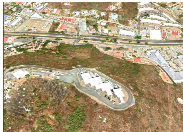
Virgin Islands Industrial Park, St. Thomas. Source: Google Earth
