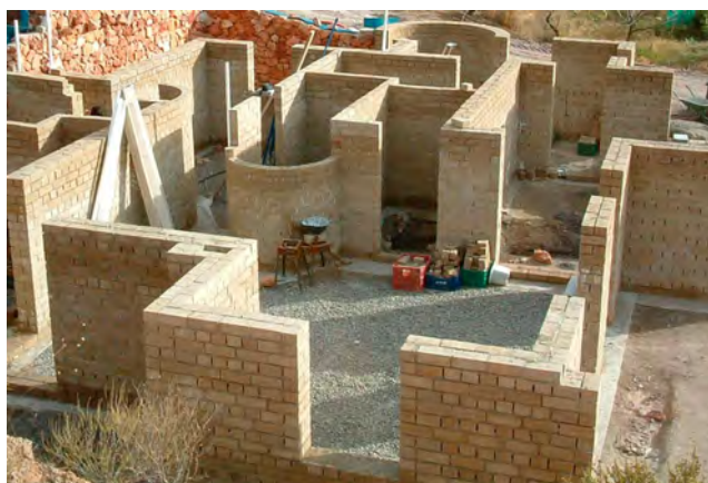
Examples of hemp building materials ("hempcrete"). Research into manufacturing applications of hemp can support research, agriculture, manufacturing, and construction industry jobs in the Territory.
