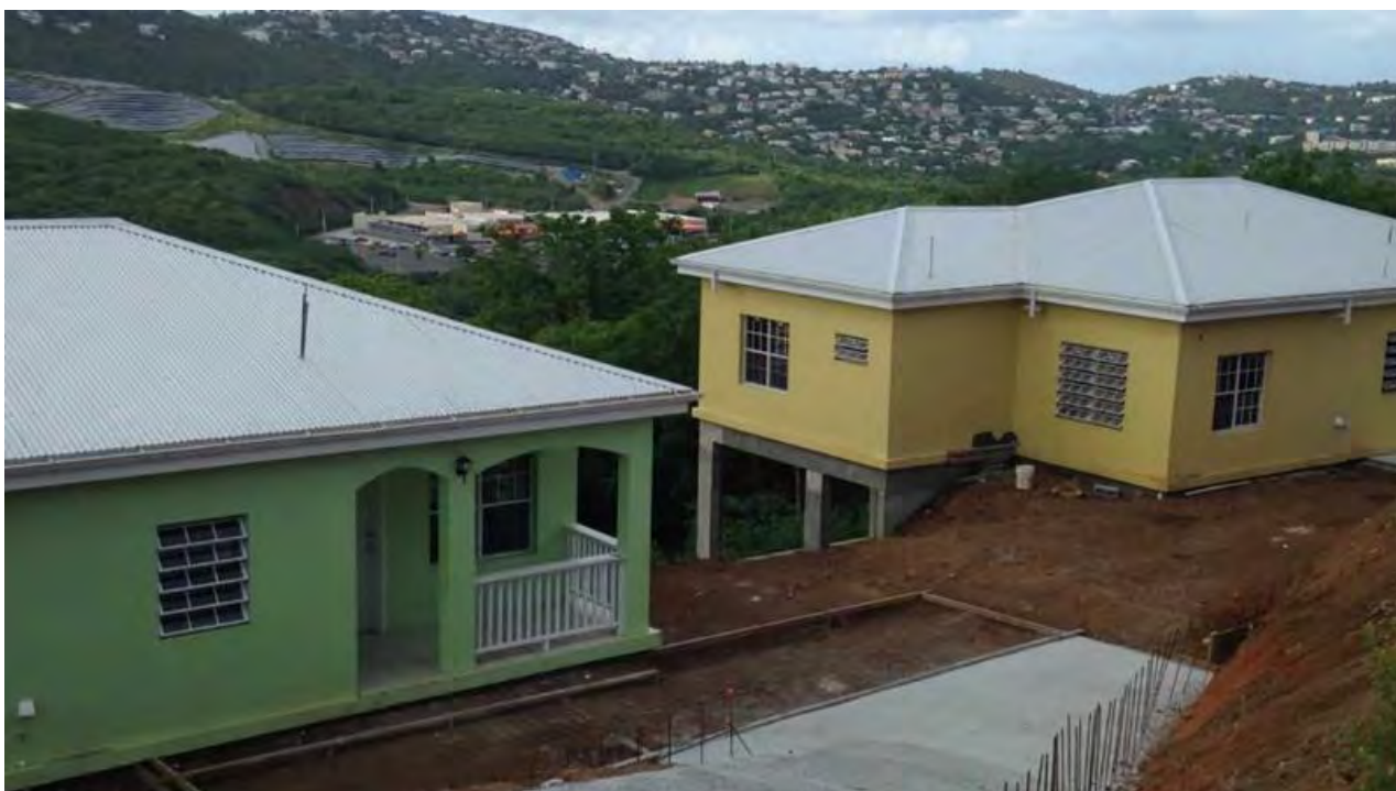
The Whispering Hills subdivision was developed by VI Housing Finance Authority in 2015 to help facilitate affordable homeownership.
